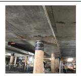
Pipework for new accessible pan is incorrectly cast-in and will clash with adjacent finishes. This causes knock-on effects to other finishes such as walls, cubicles and create risks to compliance. Identifying these early gives time to remediate.
